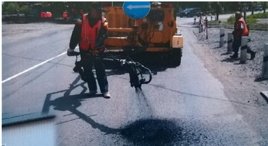
Fig. 3. Repair of pavement with injection method.
