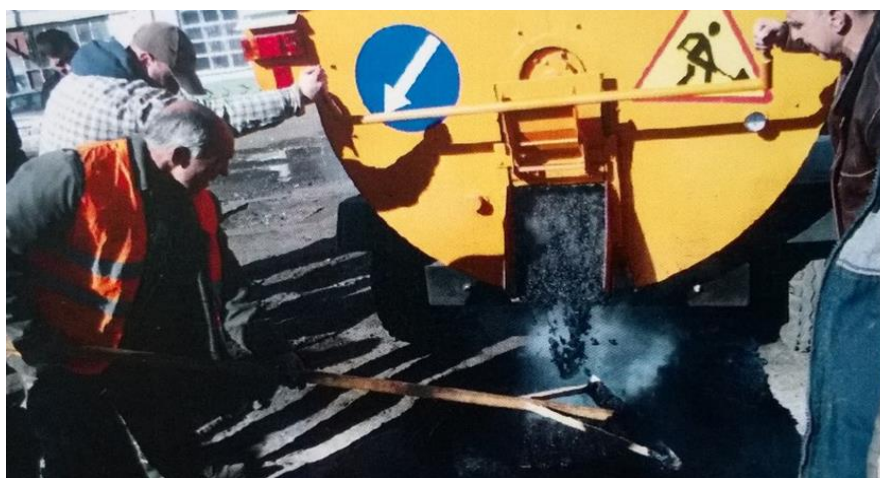
Fig. 2. Pavement repairing with cast asphalt by "recycling" road equipment.
