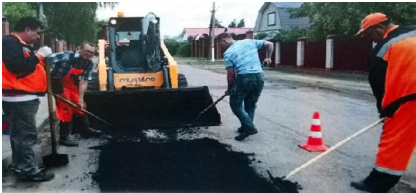
Fig. 1. Repairing of asphalt pavement using hot bituminous material.
