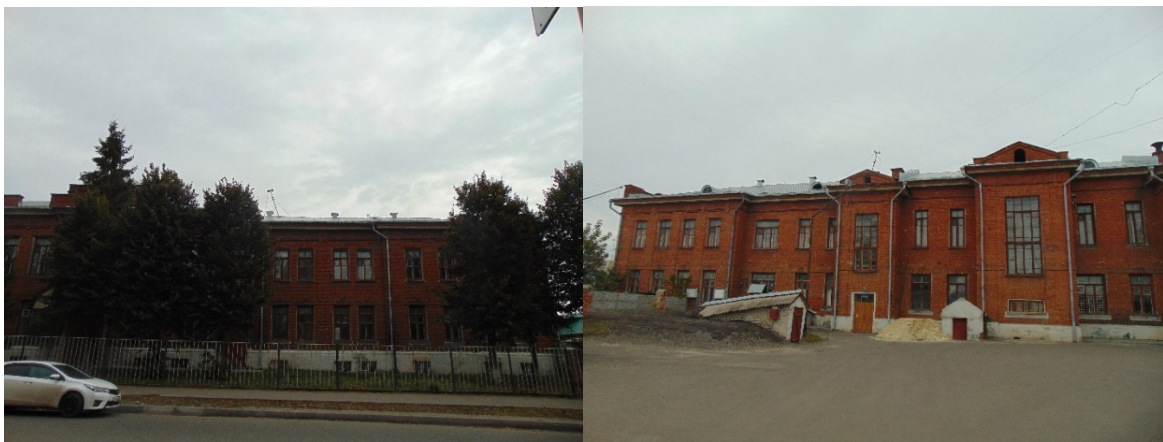
Figure 1 – The main facades of cultural heritage objects of regional significance of the “Ensemble of provincial zemsky hospital. The infectious housing” in Tambov
