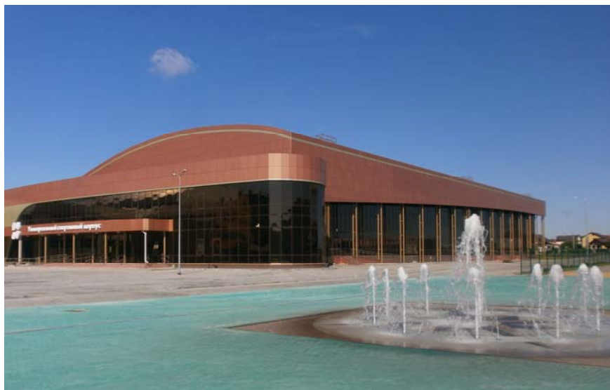
Figure 1 - Building of “Martial Arts Center”
